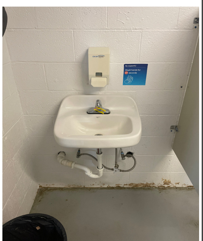
100-28 - K-12 Building - Men's Locker Room
