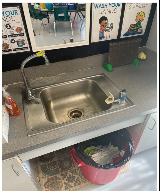
100-36 - K-12 Building - Room E9
