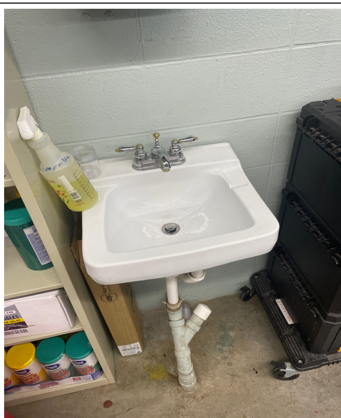
100-2 - K-12 Building - Room HS3
