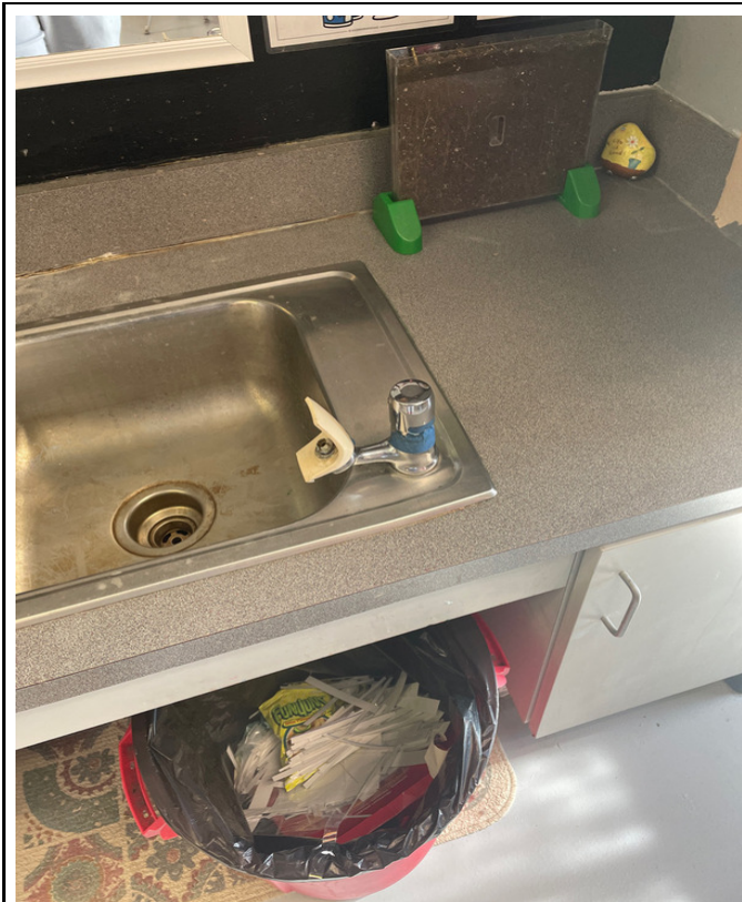
100-37 - K-12 Building - Room E9
