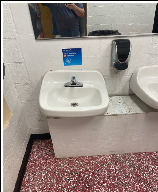
100-33 - K-12 Building - Women's Restroom East Hallway Outside of Gymnasium Left
