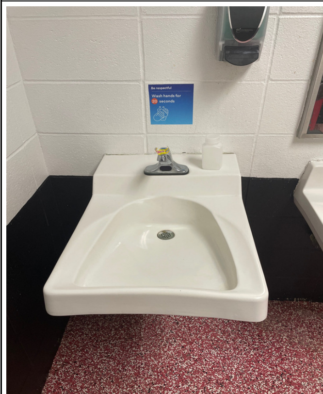
100-15 - K-12 Building - Men's Restroom Across From Library Far Left
