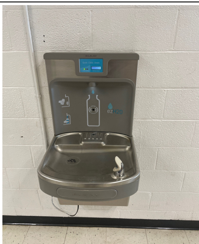
100-32 - K-12 Building - East Hallway Outside of Gymnasium
