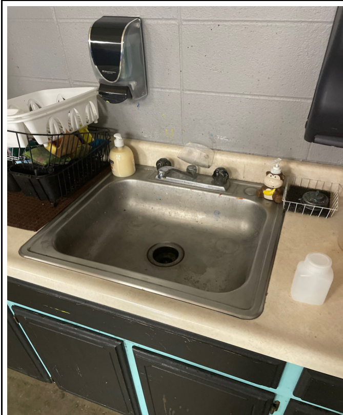
100-3 - K-12 Building - Room HS5
