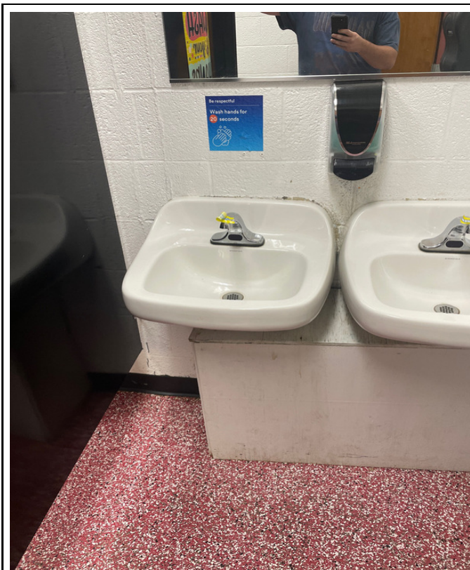
100-29 - K-12 Building - Men's Restroom East Hallway Outside of Gymnasium Left
