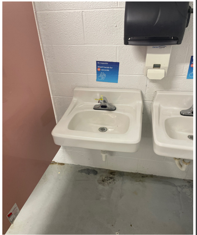
100-26 - K-12 Building - Women's Locker Room Left
