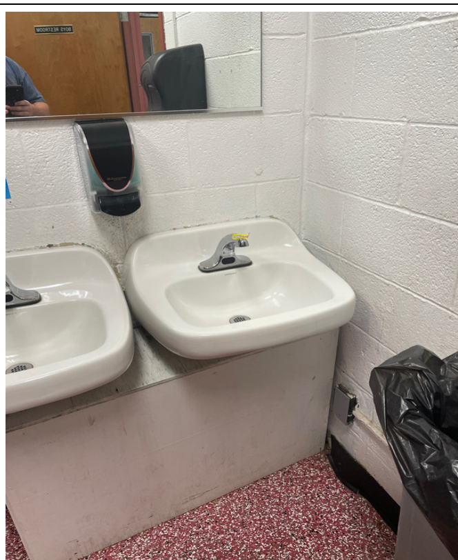
100-30 - K-12 Building - Men's Restroom East Hallway Outside of Gymnasium Right
