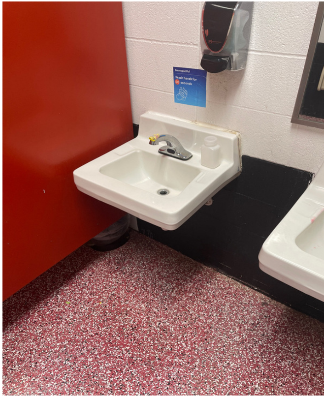
100-9 - K-12 Building - Women's Restroom Across From Library Far Left
