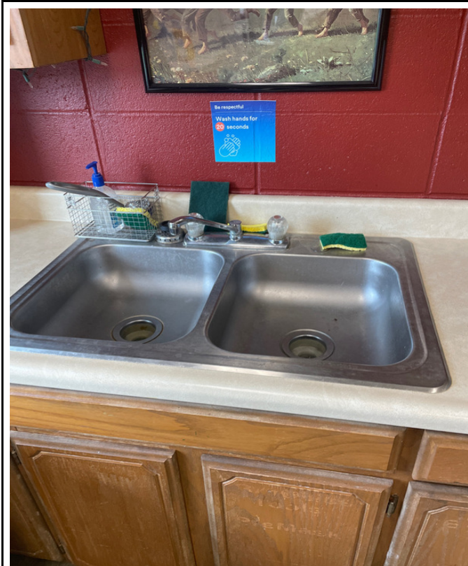
100-7 - K-12 Building - Room HS9 West Wall
