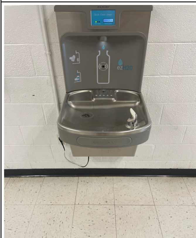
100-31 - K-12 Building - East Hallway Outside of Gymnasium
