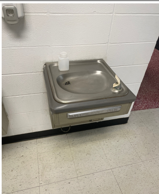
100-14 - K-12 Building - Hallway Across From Library Right
