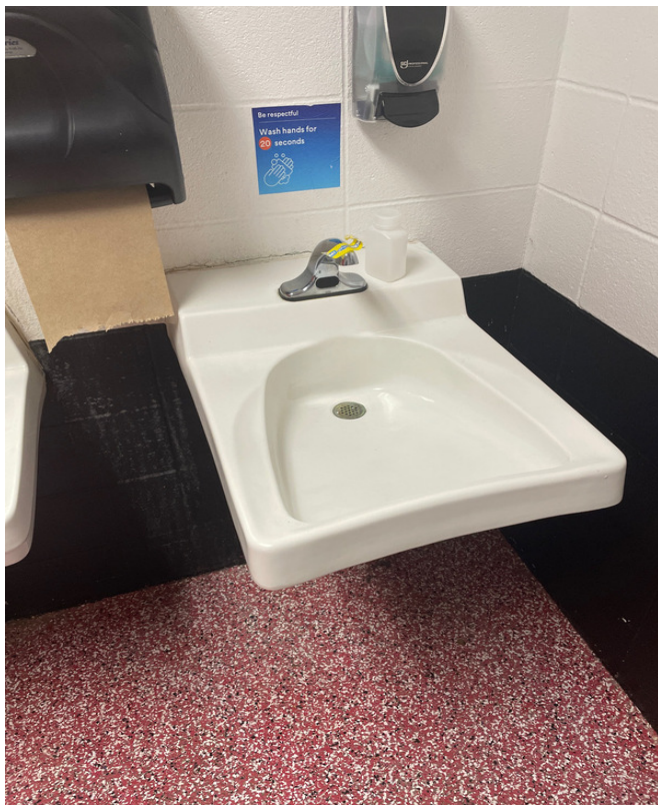
100-11 - K-12 Building - Women's Restroom Across From Library Far Right
