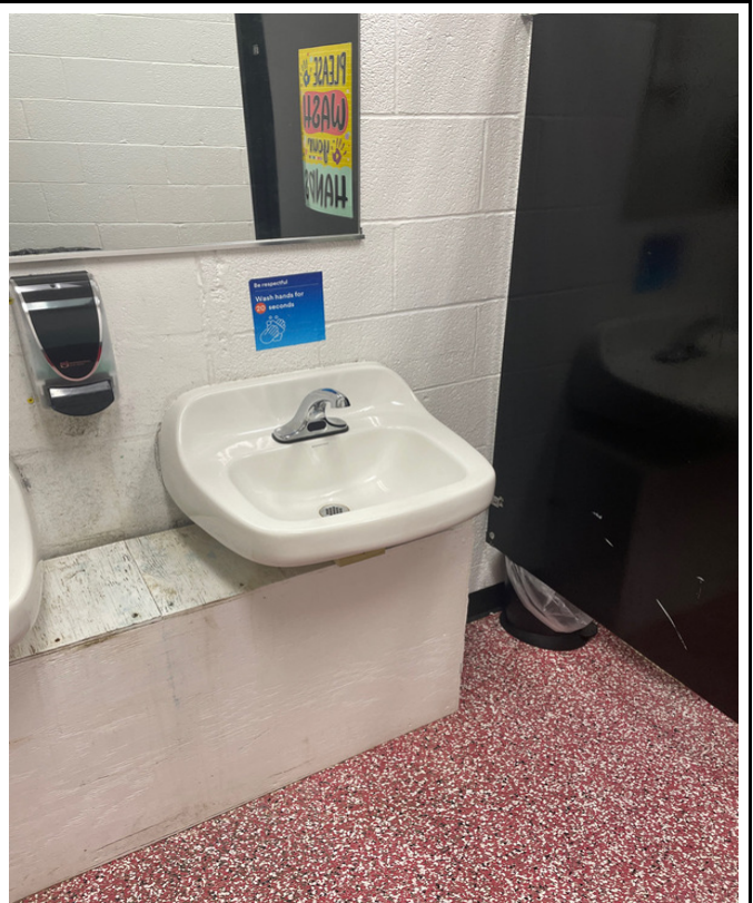
100-34 - K-12 Building - Women's Restroom East Hallway Outside of Gymnasium Right
